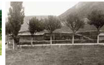
Ladestelle Perchesberg / Quai Perchesberg
